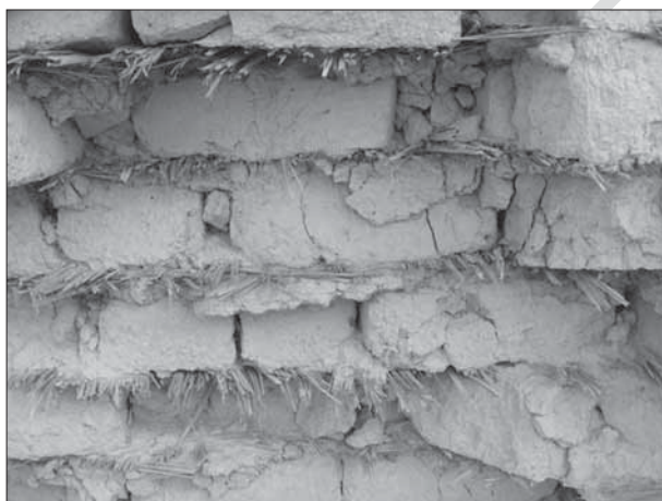
Fig. 9. Brickwork at Tell Babil with reed matting between the courses in February 2009. Photo J.E. Curtis.
